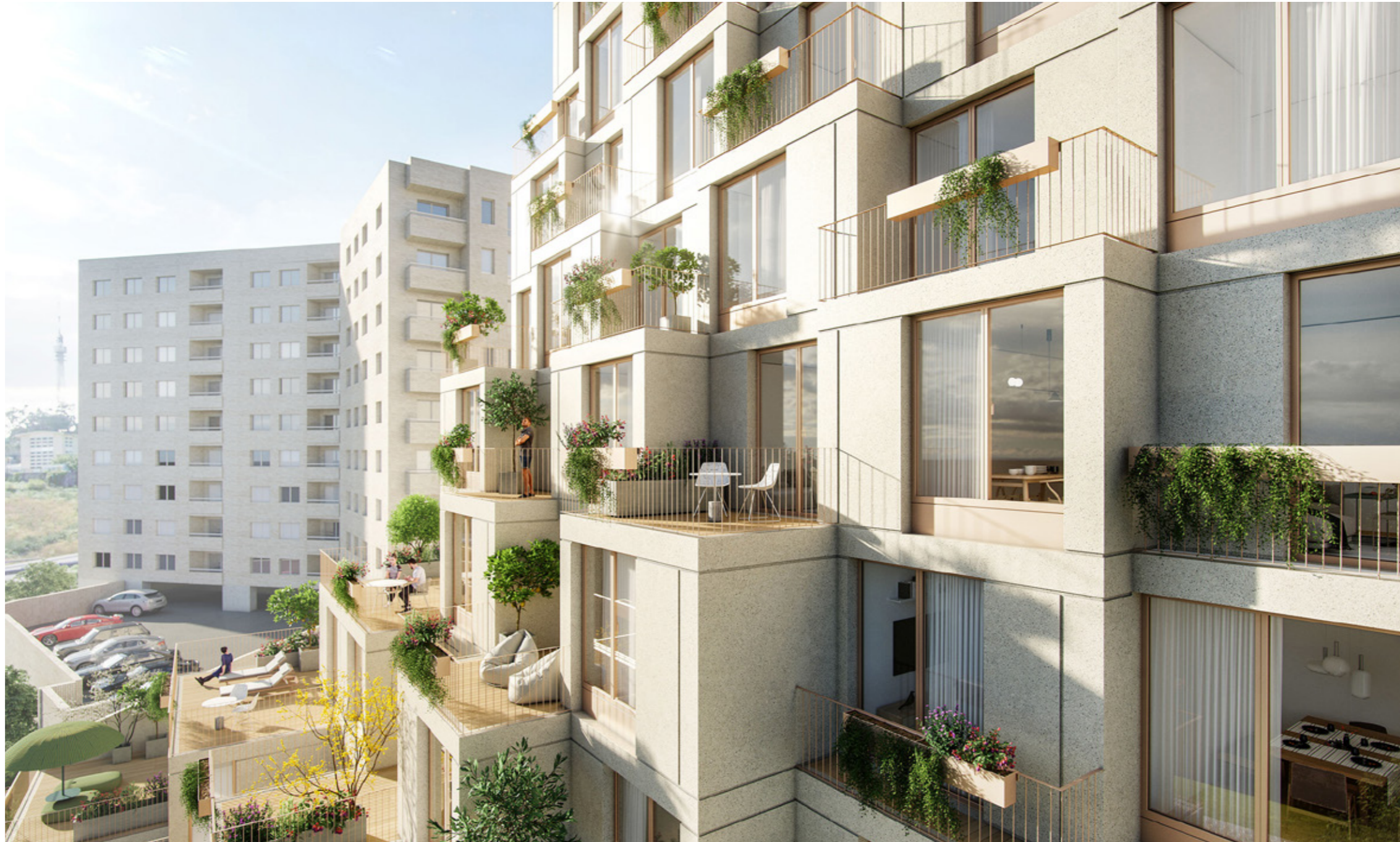
The building is designed to maximise the site's building capacity. The terraced geometry adapts itself to the plot's topography, enhancing the connection to the outside.
